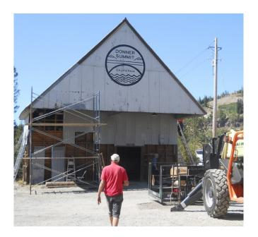
The Shed after completion of the logo painting task Friday afternoon. The forklift is at right. Scaffolding supports panel replacement on the east side, while a volunteer replaces lower roof fasteners using a ladder on the right (DSCN6445.jpg).
